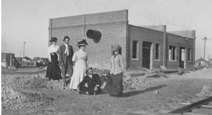
Colby's Power Plant
